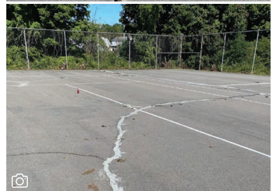
Before and After: Asphalt repairs in progress at New Britain Transitional Center.
